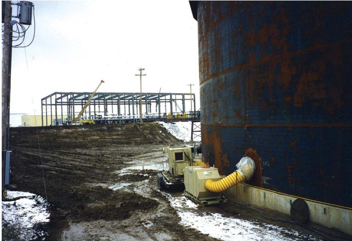
*Fig. 1: All heaters discussed here are placed outside the tank because of size constraints, fuel fumes, and other safety issues.*
